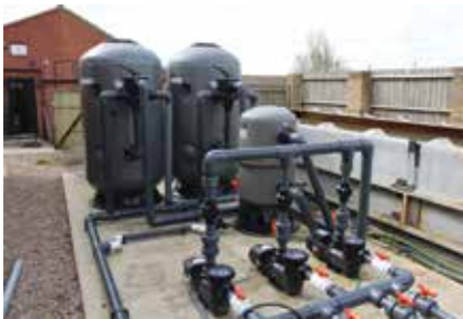
70XL Commercial MultiCyclone, two Micron SMDD 1050 fibreglass filters, three Hydrotuf pumps and glass media.
